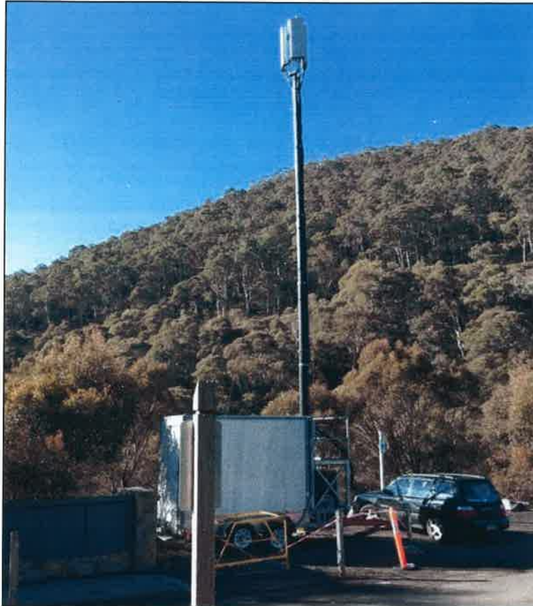
Photo 4: Temporary Cell On Wheels (COW) telecommunications facility at Thredbo Village carpark, deployed by Optus for ski season 2014.
